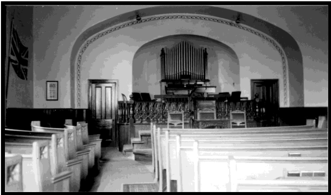
Interior of Yonge Street Building
